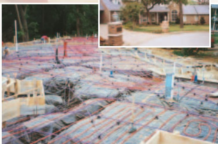
Post tension concrete slab
