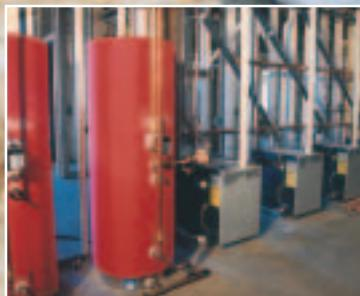
Multiple, staged boilers respond to the system's heating requirements.
