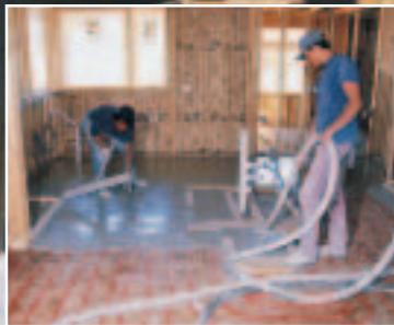
Therma-Floor® is installed to provide the ideal thermal mass.
